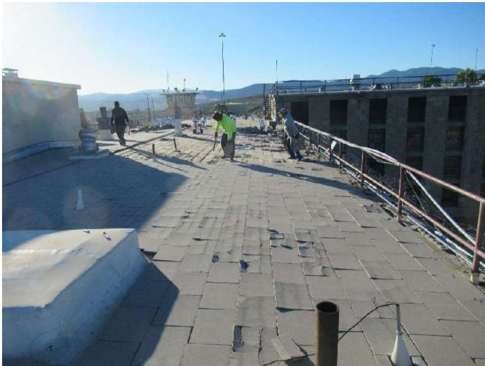
REMOVING THE CONCRETE PAVERS IN THE HEAT
