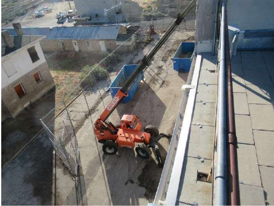
WORKERS DON'T RIDE THE LIFT; THEY CLIMB A 4-STORY LADDER
