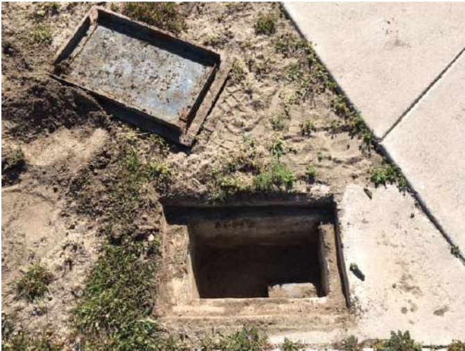
DRAINS ARE CLEAR
